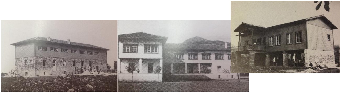
Figure 7. Grand school building and teacher houses
